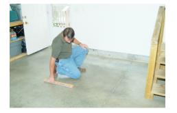
Note; It will ease the installation by putting ¼" shim stock under the shelter walls to allow your pry bar to maneuver the walls in place. Once walls have been moved and are in position, remove shims.
