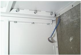
Remove all shims and test door opening & closing, adjust door so it clears floor by 1/8" and does not drag against the floor.
