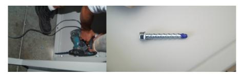
Insert the rear concrete anchor Wedge Bolts illustration # 5 and tighten evenly "do not over tighten" With the shelter fully open locate & drill the holes for front anchors using 5/8" concrete bit and hammer drill. Insert the front concrete anchors and tighten evenly "do not over tighten". Clean area after drilling to remove concrete dust and debris.
